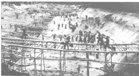
An open-cast tin mine
